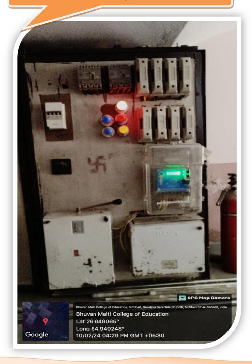
This is Electricity Borad installed in College Reception Area for the purpose of Control alternate source of energy.
